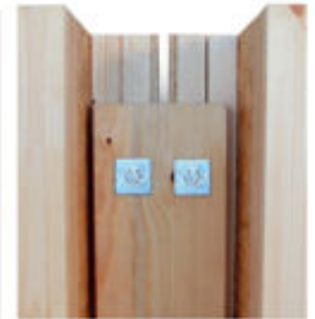
Example of dismantlable wood structure. (GXN)
